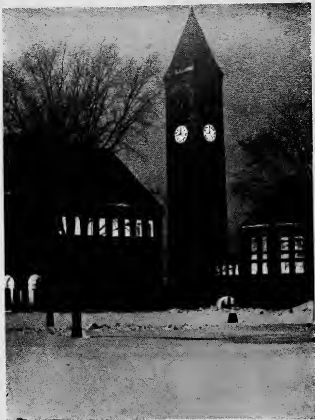
THE LIBRARY TOWER AT NIGHT
